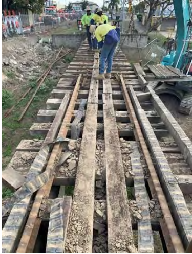
Figure 49: Dismantling work in progress (Bligh Tanner 2022)
