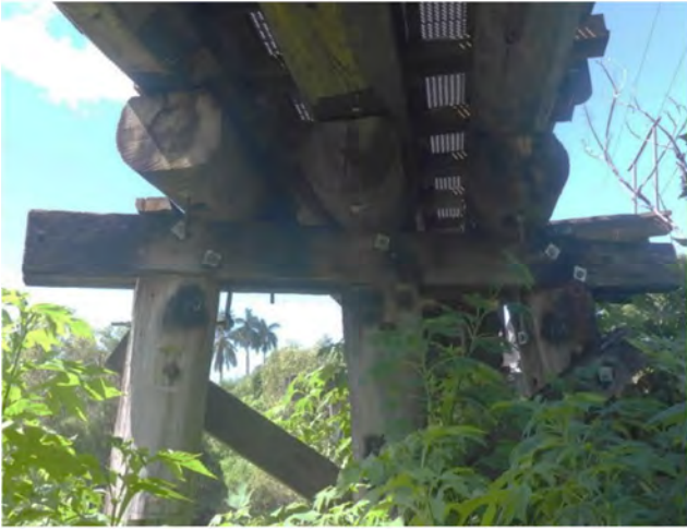
Photo 33 General view pier 3 corbels/headstock
