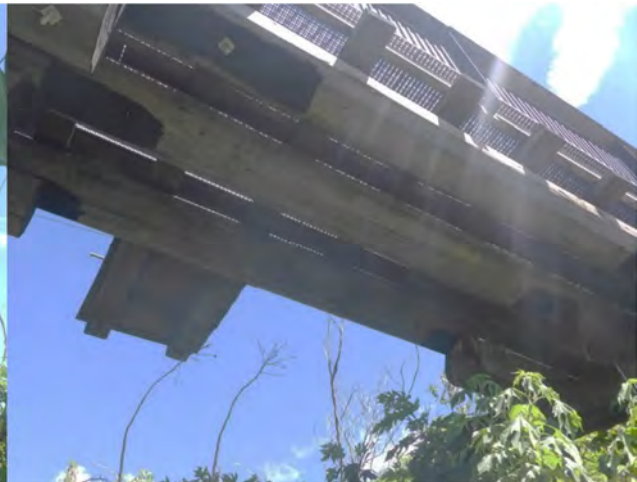
Photo 48 General view span 4 girders
