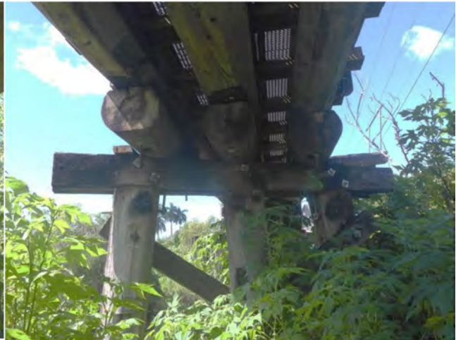
Photo 6 General view of pier 3
