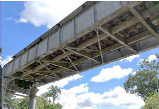
Photo 50 General view span 6 girders
