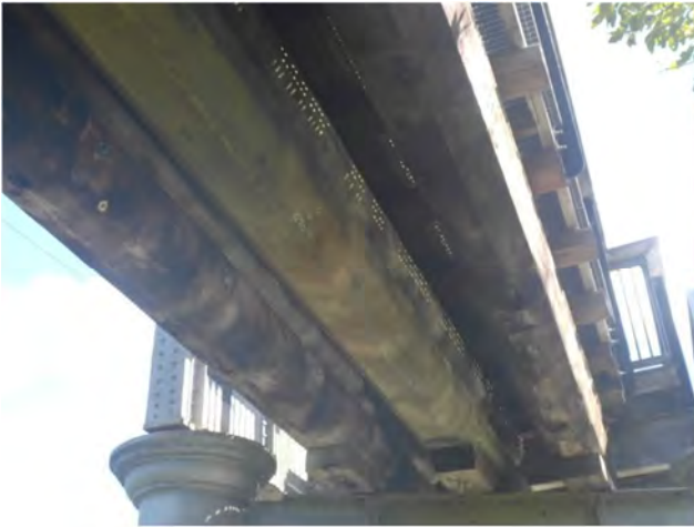
Photo 61 General view span 7 girders
