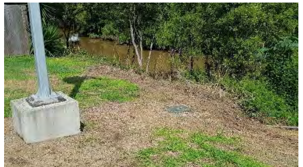
Figure 73: Slashed area around monitoring station on SE embankment (Converge 2022).
