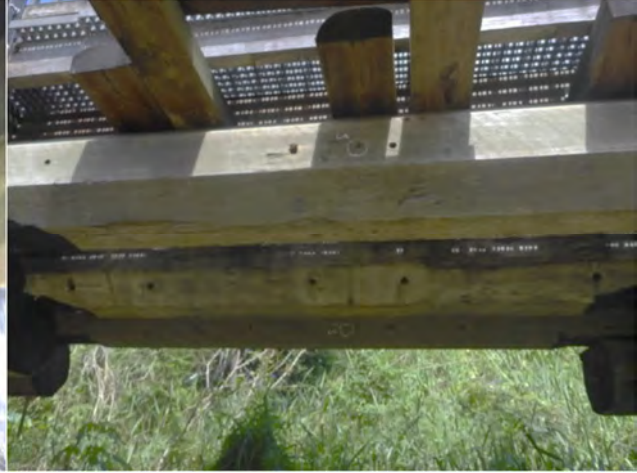
Photo 46 General view span 2 girders
