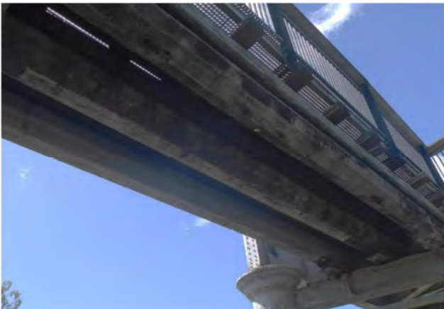
Photo 49 General view span 5 girders
