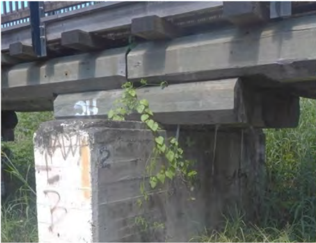
Photo 31 General view pier 1 corbels
