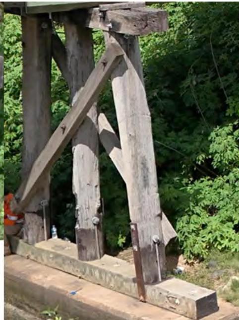
Photo 8 General view of pier 4
