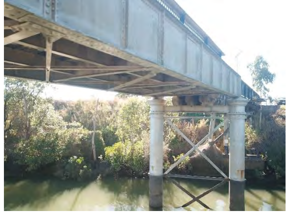
Figure 93: Span 6 and pier 7 (Converge 2020).
