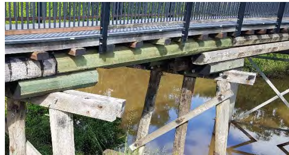
Figure 114: View of path constructed over railway line (Converge 2022).
