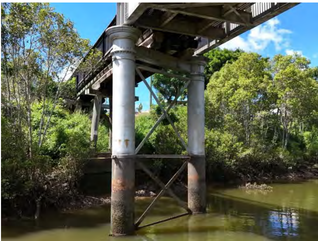
Photo 19 General view of pier 6
