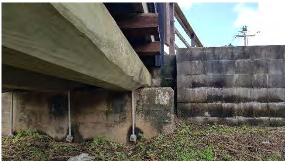
Figure 109: Pier 11 – east abutment (Converge 2022).
