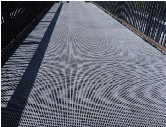
Photo 71 FRP footway sound
