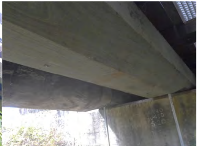
Photo 64 General view span 10 girders
