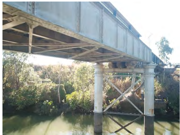
Figure 30: Span 6 and pier 7 (Converge 2020).
