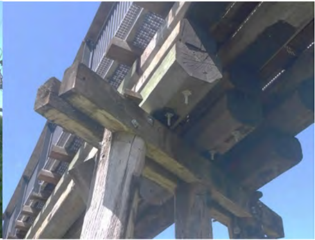
Photo 34 General view pier 4 corbels/headstock
