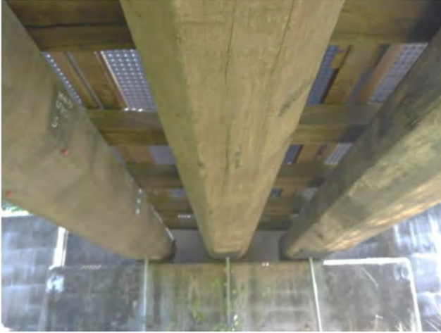
Photo 45 General view span 1 girders
