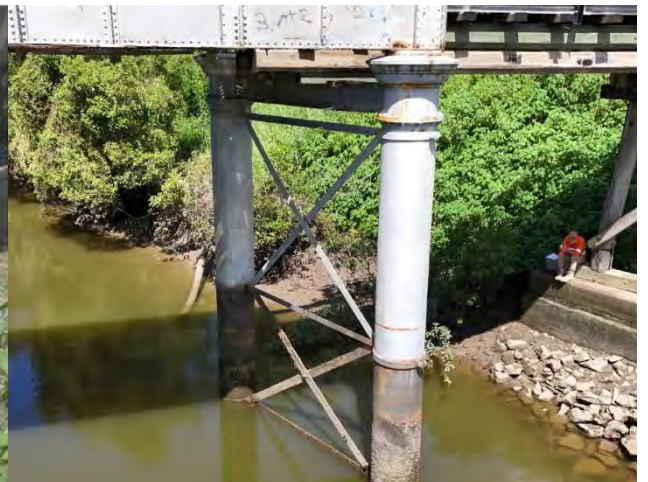
Photo 14 General view of pier 5
