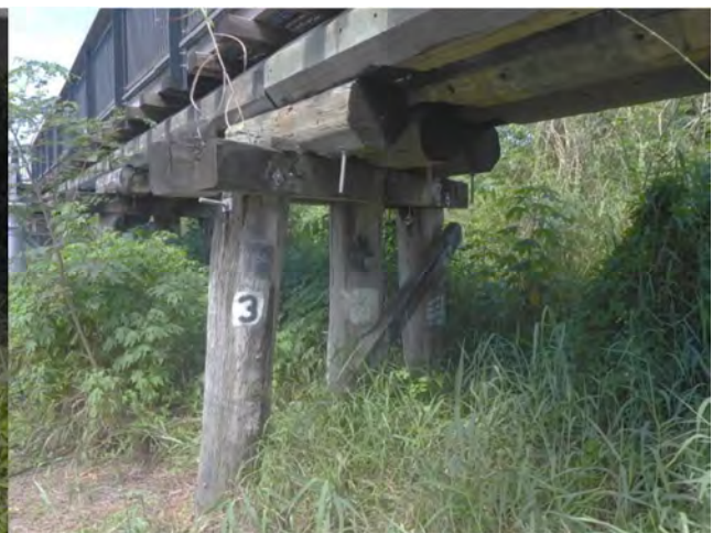
Photo 4 General view of pier 2
