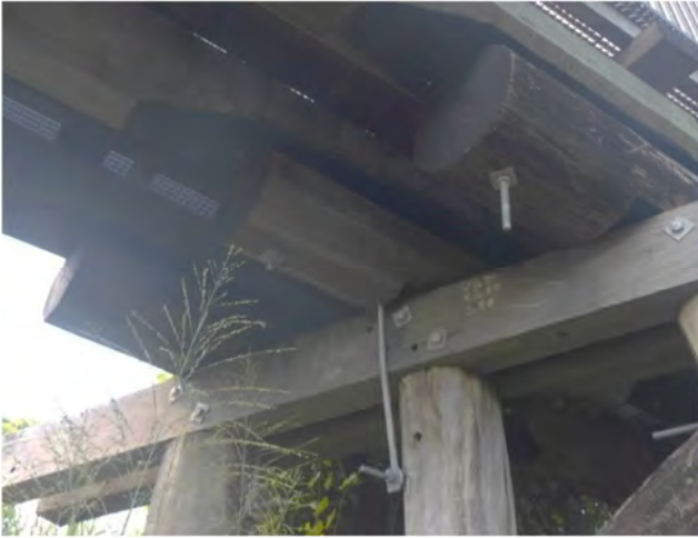
Photo 39 General view pier 8 corbels/headstock
