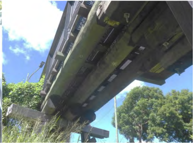
Photo 62 General view span 8 girders
