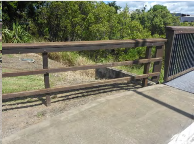
Photo 75 Approach 2 railings sound
