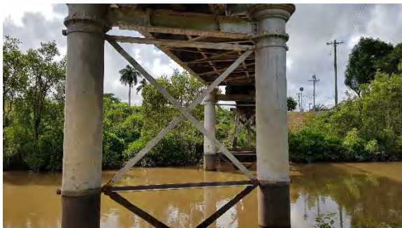
Figure 72: View to east embankment (Converge 2022).
