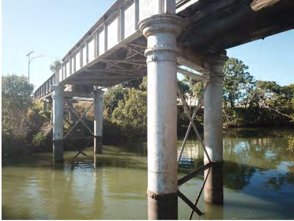
Figure 92: Pier 6 and 7 (Converge 2020).
