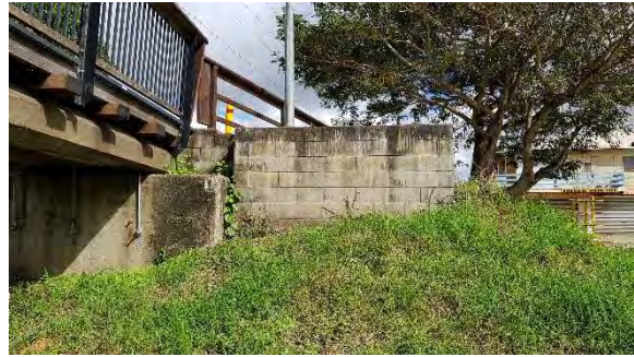
Figure 75: Short retaining wall on the NW side (Converge 2022).
