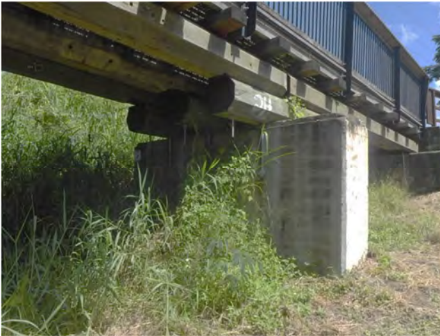
Photo 1 General view of pier 1 (1)
