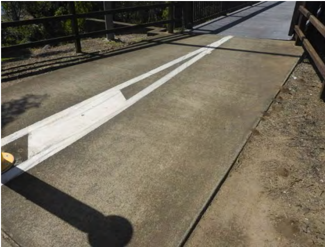
Photo 69 Approach 1 footway sound
