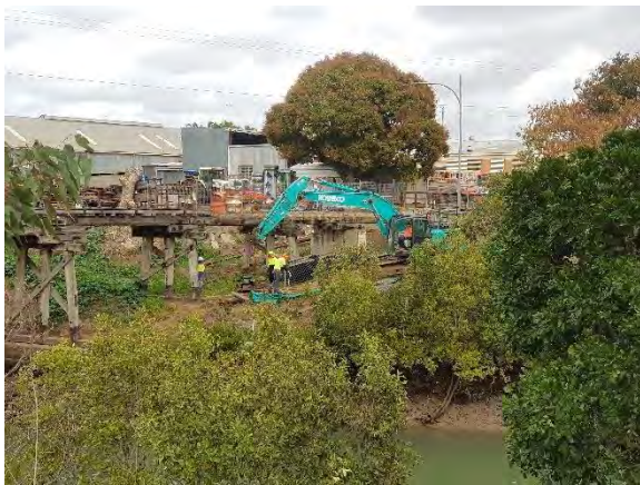
Figure 47: Stage 1 work in progress in September 2021 (Converge 2021).
