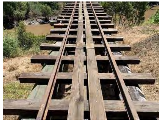
Figure 55: Replacement timber sleepers (Bligh Tanner 2022).
