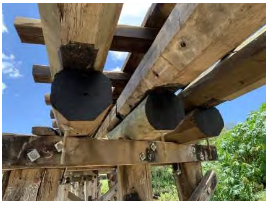
Figure 54: Replacement girder, corbel, and headstock (Bligh Tanner 2022).
