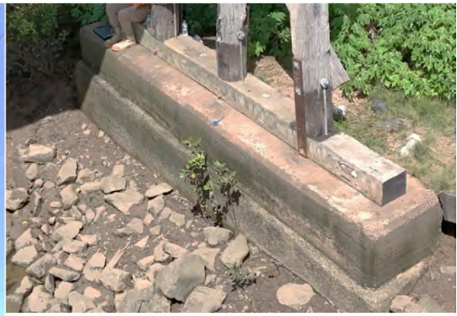
Photo 12 General view of pier 4 mass concrete footing
