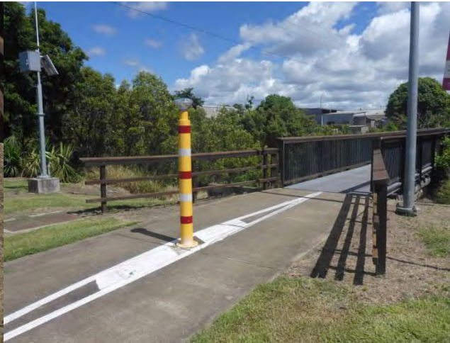
Photo 70 Approach 2 footway sound
