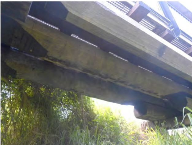
Photo 63 General view span 9 girders
