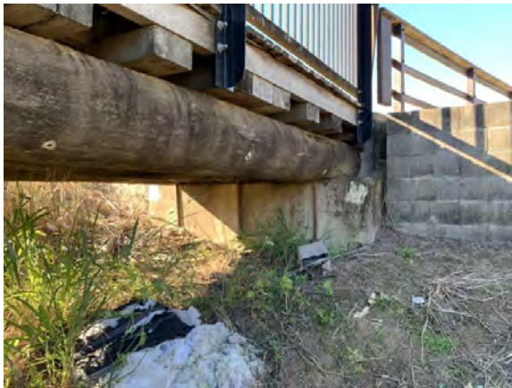
Figure 45: Pier 11 – east abutment (Bligh Tanner 2020).
