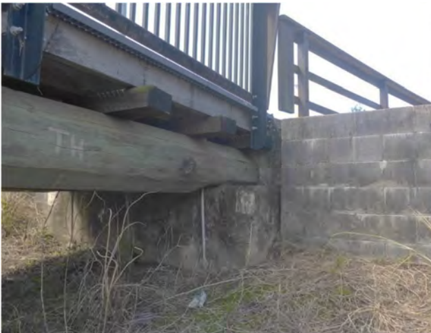
Photo 43 General view abutment 2 wall (1)
