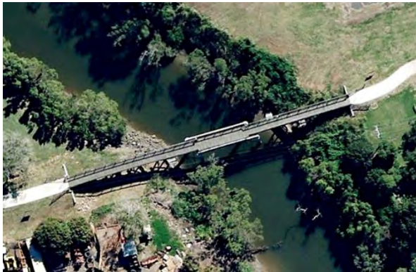
Figure 7: 2008 imagery of the Bridge (Google Earth Pro 2024).
