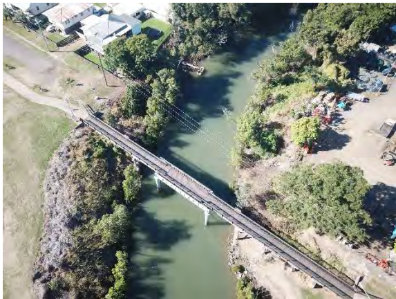
Figure 58: Aerial view of bridge (Converge 2020).
