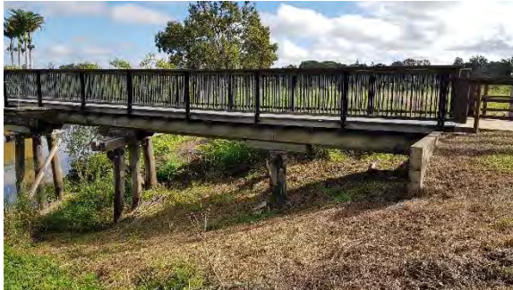
Figure 101: East bank, south side (Converge 2022).
