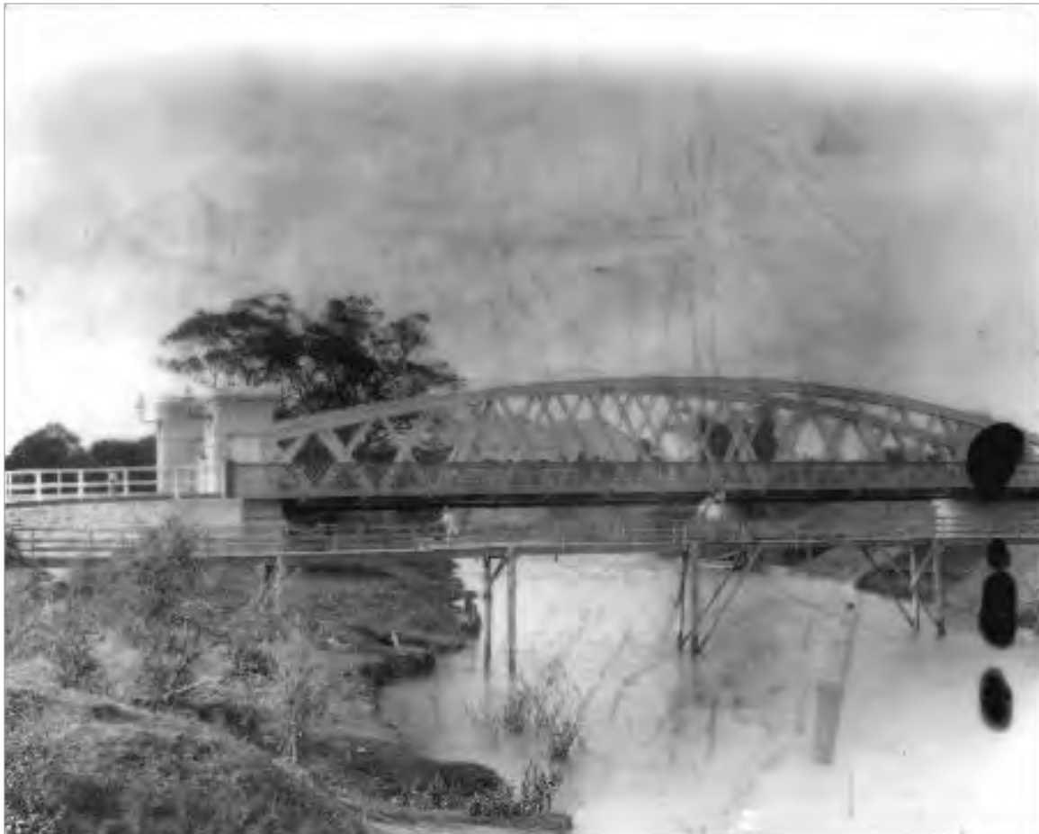
Figure 3: Old and new Kennedy Bridge over Saltwater Creek, 1899 (Picture Bundaberg Ref#01074).
