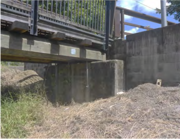
Photo 41 General view abutment 1 wall (1)
