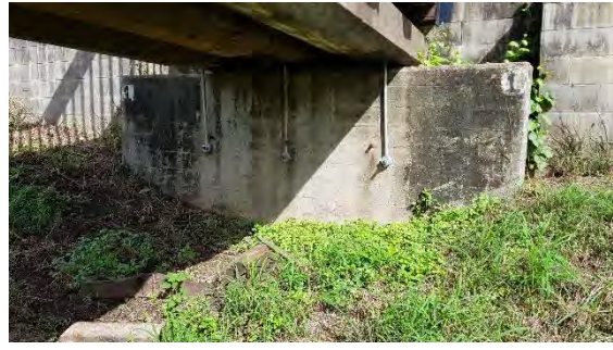
Figure 82: West abutment (Converge 2022).
