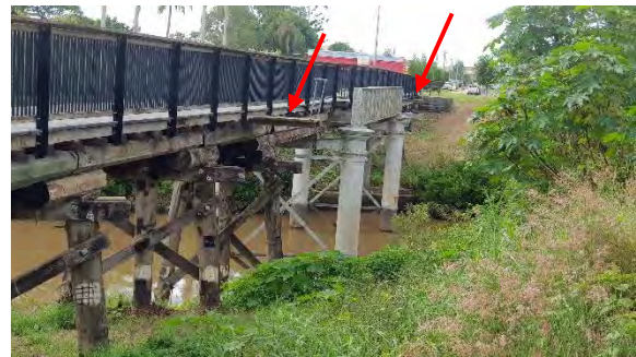
Figure 80: Southside of bridge, arrows mark platforms at Span#5 and 9 (Converge 2022).
