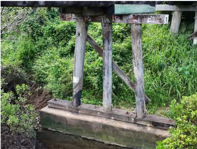
Photo 23 General view of pier 7
