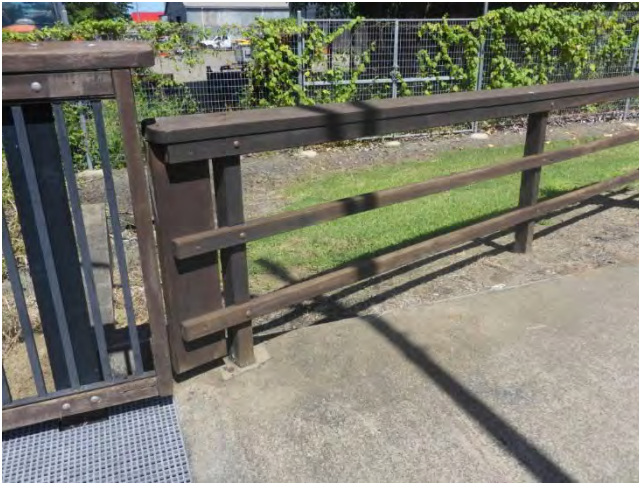
Photo 74 Approach 1 railings sound
