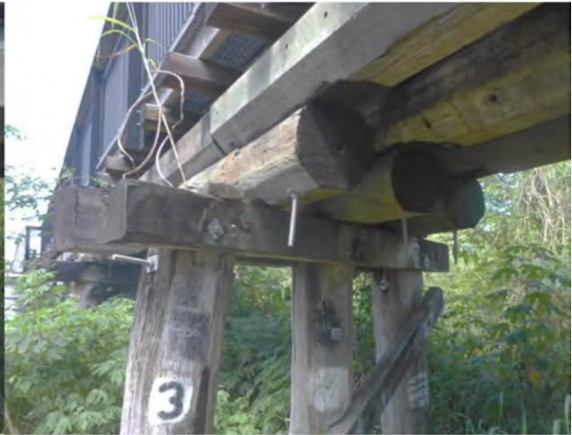
Photo 32 General view pier 2 corbels/headstock
