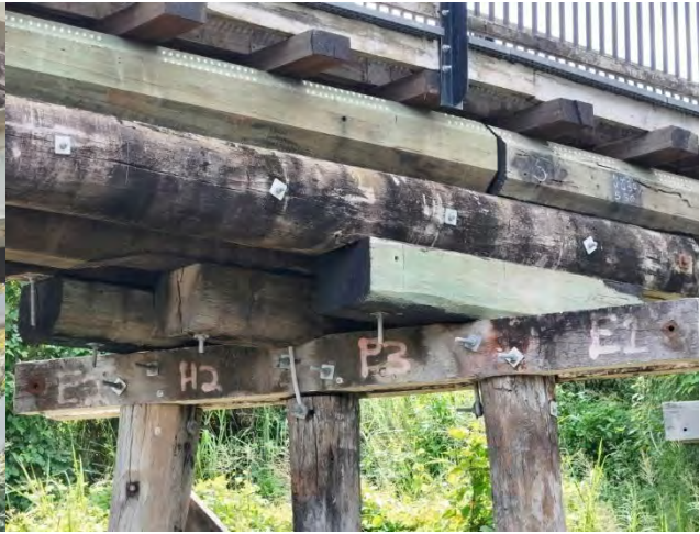
Photo 38 General view pier 7 corbels/headstock
