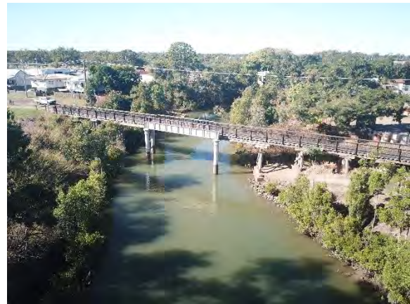
Figure 59: View south to bridge from Burnett River (Converge 2020).
