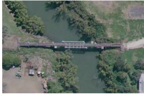
Figure 6: 2006 imagery of the Bridge, just prior to its conversion (Google Ea 2022)
