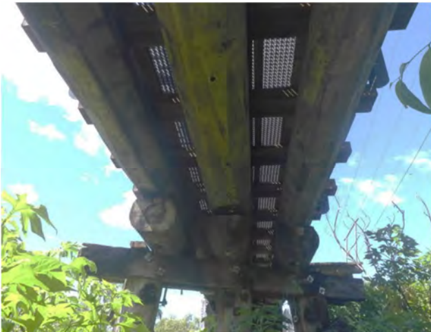
Photo 47 General view span 3 girders
