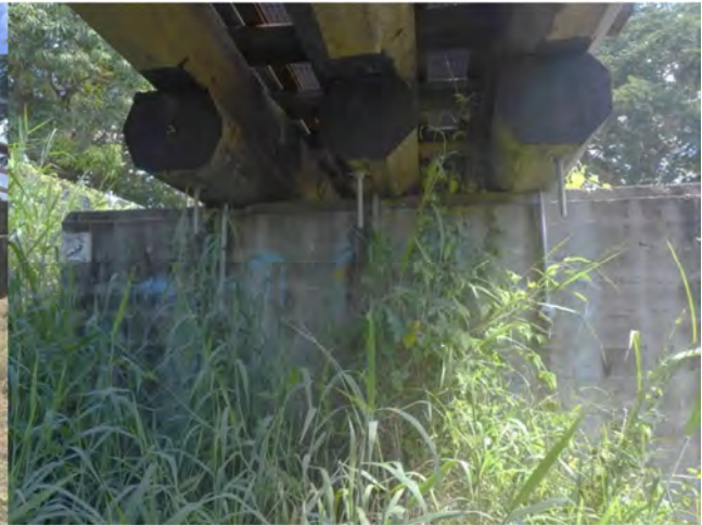
Photo 2 General view of pier 1 (2)
