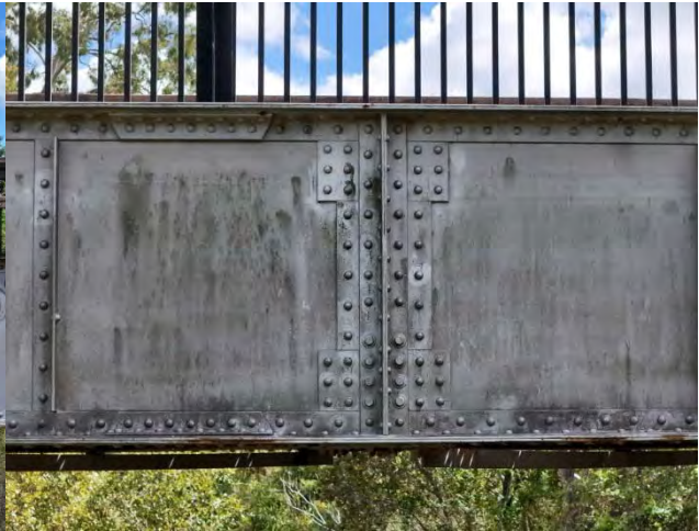
Photo 52 General view of span 6 main girders right hand side
