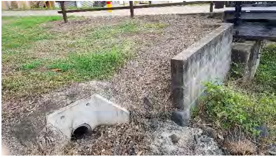
Figure 81: West termination (Converge 2022).
