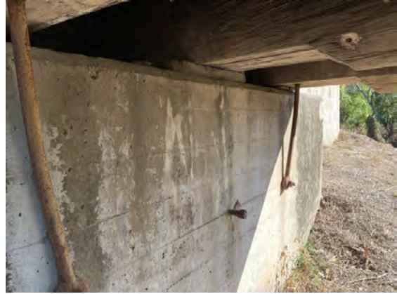
Figure 20: West abutment (Bligh Tanner 2020).
