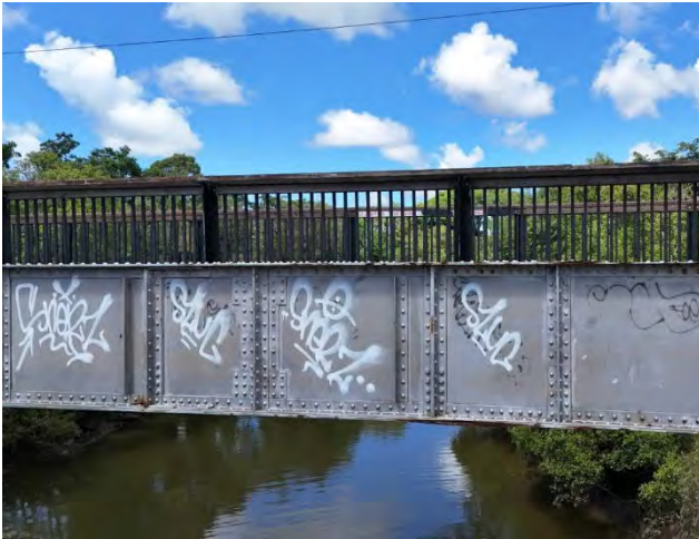
Photo 51 General view of span 6 main girders left hand side
