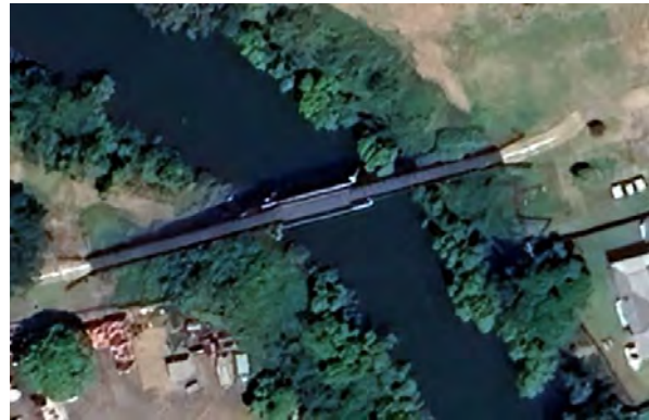
Figure 8: 2023 imagery of the Bridge (Google Earth Pro 2024).
