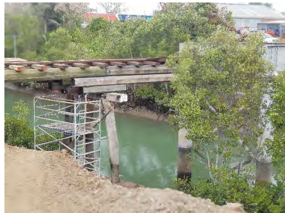
Figure 48: Stage 1 work in progress in September 2021 (Converge 2021).
