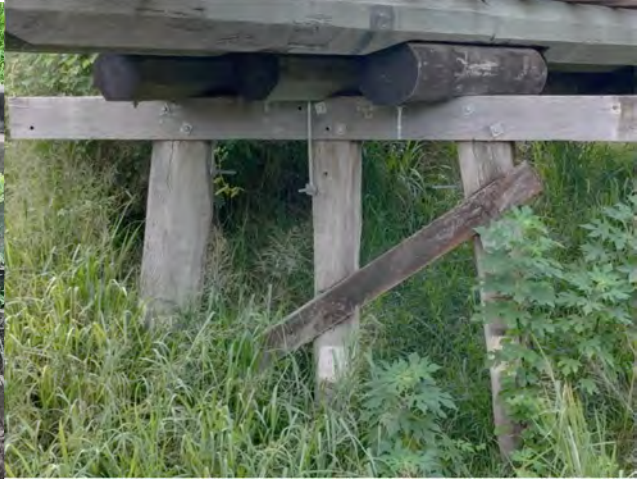
Photo 28 General view of pier 8
