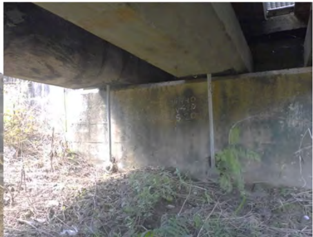
Photo 44 General view abutment 2 wall (2)
