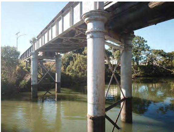
Figure 29: Pier 6 and 7 (Converge 2020).
