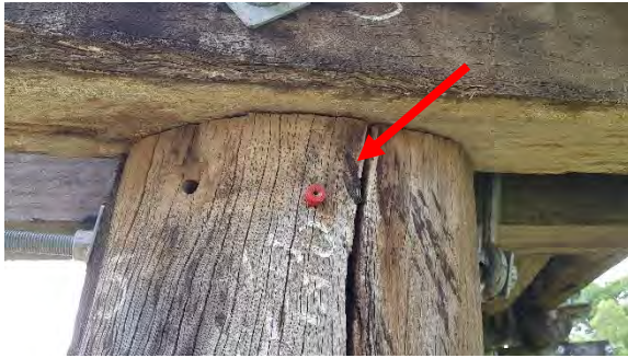
Figure 111: Cap visible on timber pier indicating pest/fungal treatment (Converge 2022).
