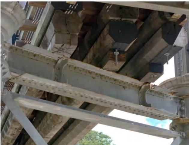
Photo 35 General view pier 5 cross beam
