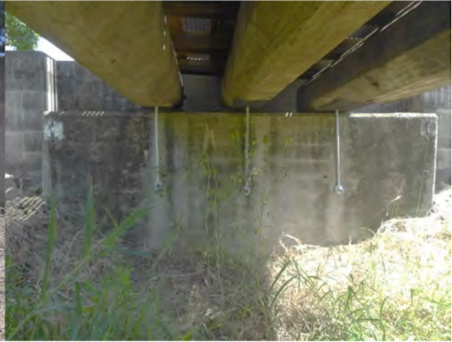
Photo 42 General view abutment 1 wall (2)
