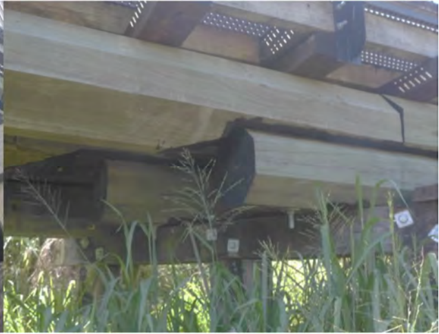
Photo 40 General view pier 9 corbels/headstock
