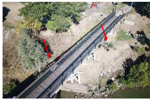
Figure 18: West bank, arrows mark platforms at Pier#3 and 5 (Converge 2020).
