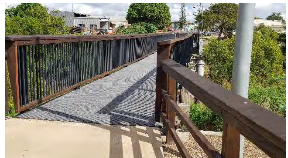
Figure 116: Approach on east side (Converge 2022).
