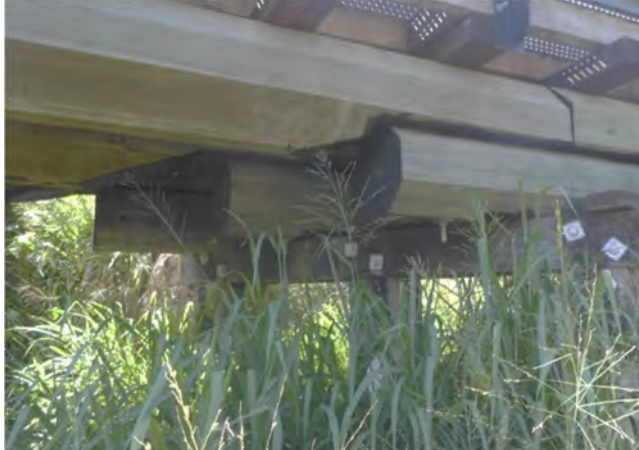
Photo 30 General view of pier 9
