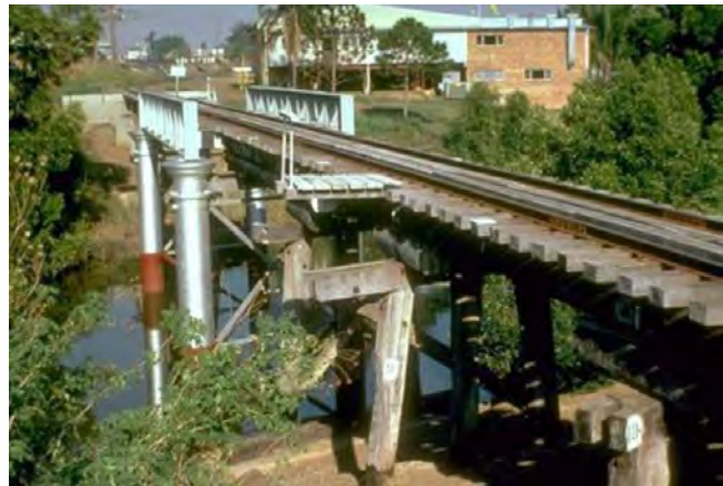
Figure 4: Saltwater Creek Railway Bridge, date unknown (Converge 2022).
