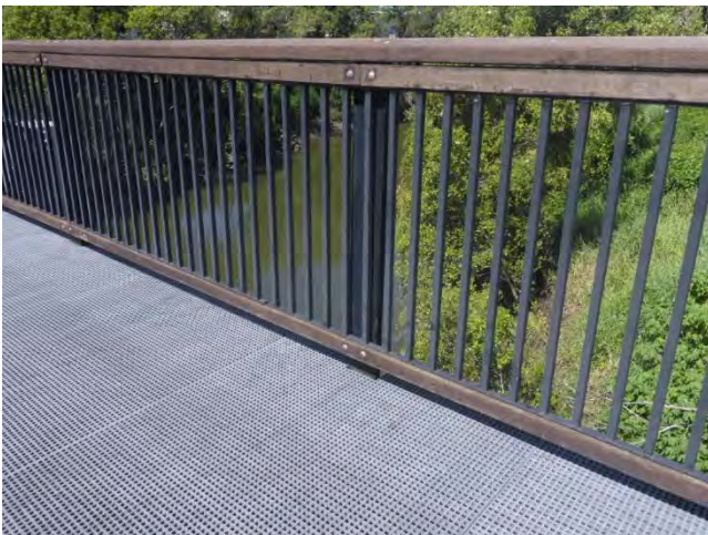
Photo 76 Bridge railing sound
