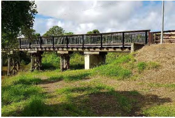
Figure 68: View to NW embankment (Converge 2022).
