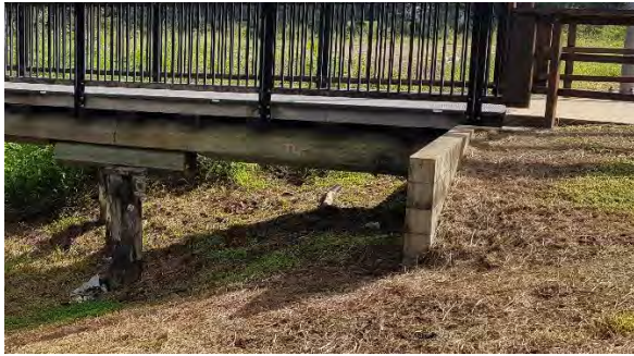
Figure 74: Short retaining wall on the SE side (Converge 2022).
