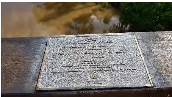
Figure 115: Plaque fixed to handrail (Converge 2022).
