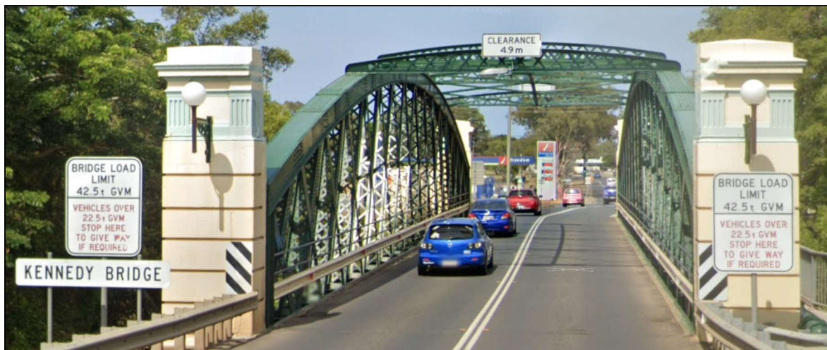
Figure 21: Kennedy Bridge Heavy Vehicle Restrictions (Google Street View 2020)
