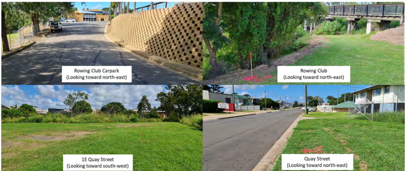
Figure 2-2: City Levee Alignment Site
